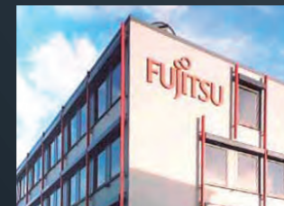
R&D Center in Fujitsu General (EURO) GmbH (Germany)
